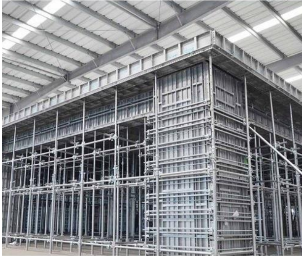
Figure 1. Aluminum formwork system.
