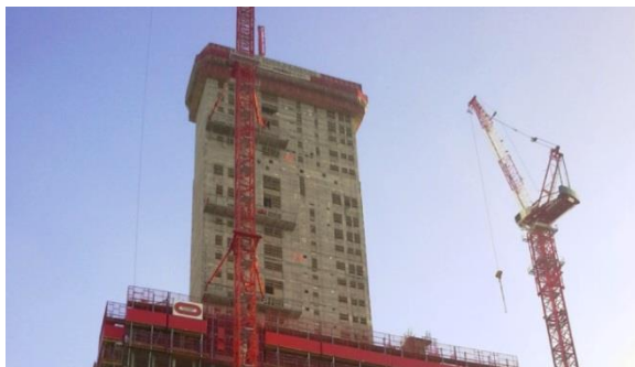
Figure 3. Slip formwork system.
