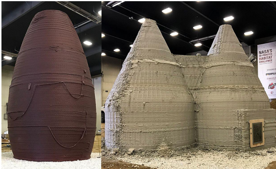
Figure 1. One-third-scale 3D printed Martian habitats constructed during Phase III of NASA’s 3D-Printed Habitat Challenge: MARSHA (left) by AI SpaceFactory and Den@Mars (right) by Penn State (source: Staedter [5]).
